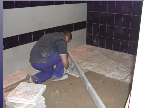
Flooring and tiling
