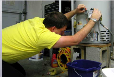
Maintaining thermal and fluids installations
